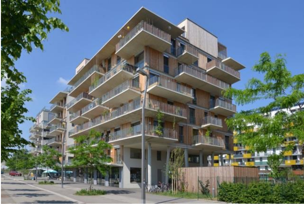
6.17: Housing Complex in Bednar Park, Vienna - subsidized home with 39 residential units, 500m 2 common rooms and 400m 2 commercial units, winning project for the Nordbahnhof developer competition, planning period 2010–2013 and completion end of 2013, designed by Einszueins Architektur © MA19
