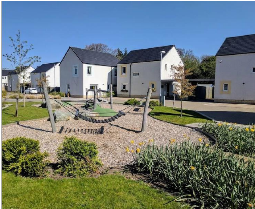
5.35: The Scottish Government worked with house-builder Mactaggart and Mickel to demonstrate how 'Designing Streets' policy could be applied on an exemplar residential development in East Renfrewshire, Eaglesham, Scotland, design by Proctor & Matthews Architects, 2011 ©Kristen Anderson
