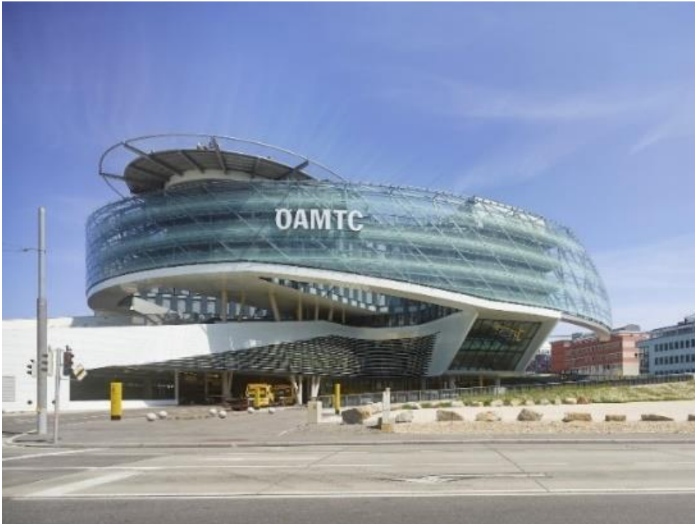
6.17: The headquarters of the Austrian Automobile, Motorcycle and Touring Club (ÖAMTC) in Vienna, from Pichler & Traupmann Architekten (2016), was the result of a design competition held in 2013, organised by the Austrian Chamber of Architects with the participation of the City Council © Roland Halbe
