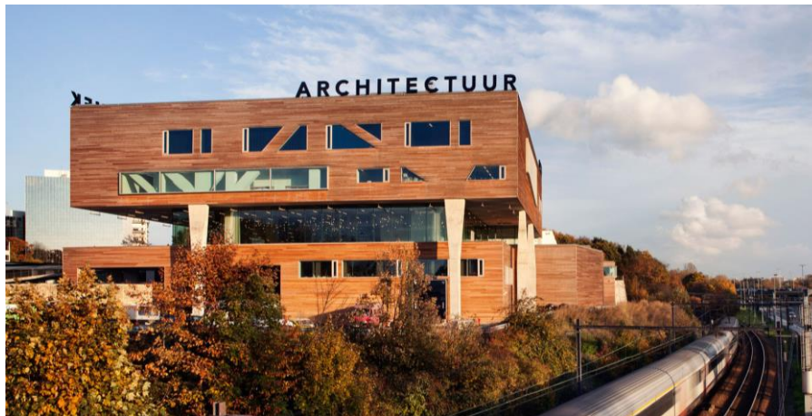
5.1: The new wing of the International Arts Centre 'DeSingel', where the Flanders Architecture Institute (VAI) is based since 2001, designed by Stephane Beel Architects, Antwerp, Belgium © EI
