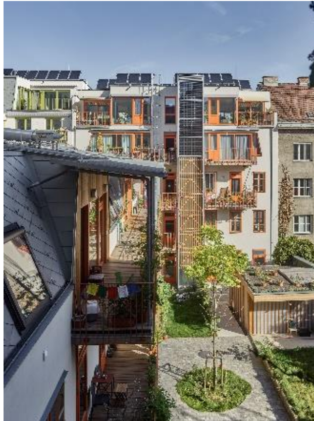
6.15: Smart block Geblergasse, in Vienna, designed by Zeininger Architekten Technical (2021), was awarded the State Prize for Architecture and Sustainability. The block comprises almost 20 plots. The existing houses were expanded, raised, and renovated, and for the first time in Austria, geothermal energy was used in historic buildings ©BMK/Kurt Hoerbst
