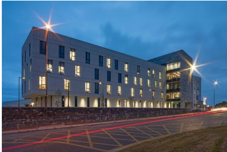
5.16: Galway Regional Garda (Police) Headquarters, designed by OPW Architects, in Galway, Ireland, 2018 © Kelvin Gilmore
